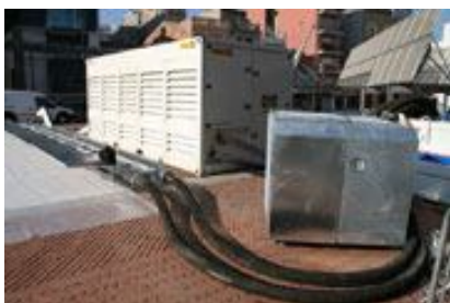
Chiller connected to an ice rink
