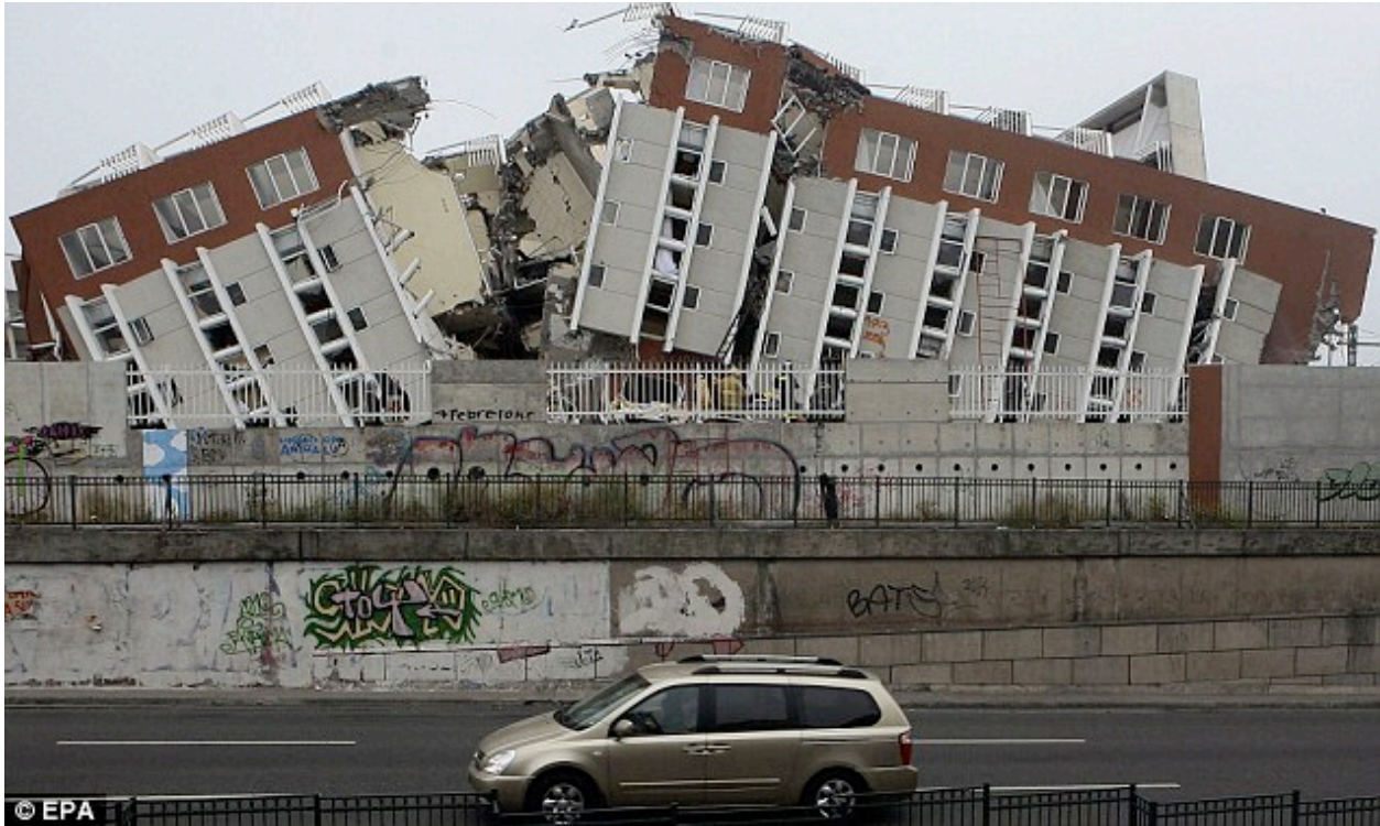
A destroyed building in Concepcion, Chile. The whole city shifted 10 feet to the west as a result of the February earthquake
