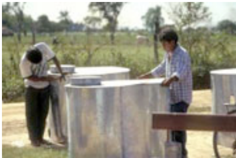
Making metal silos for grain storage
